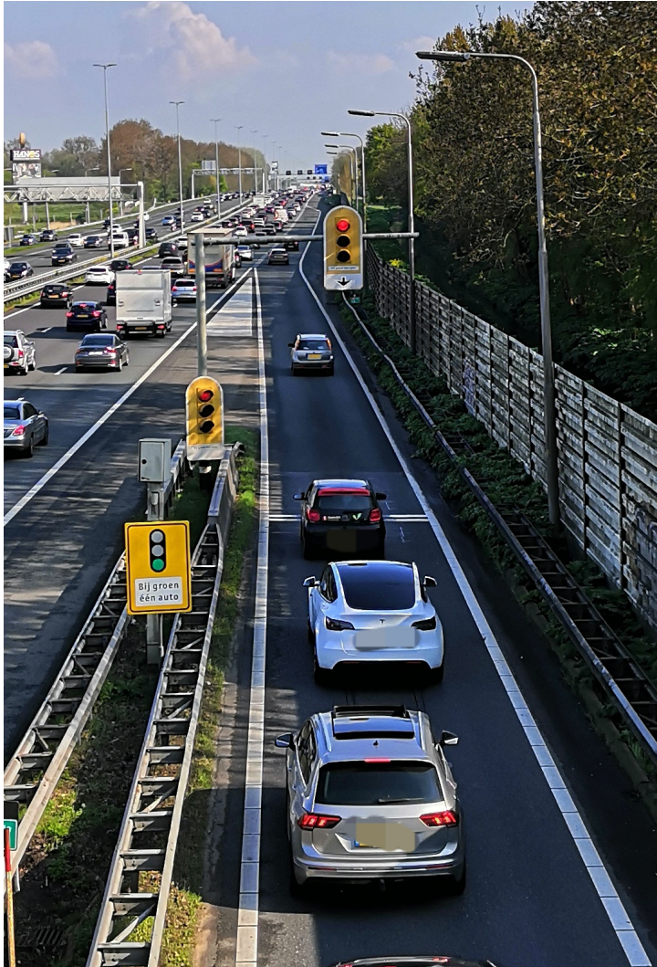
Figure 1.2: Ramp metering at the A13 freeway, Delft, The Netherlands.
