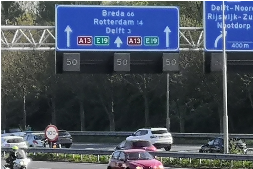
Figure 1.1: Variable speed limits signs along the A13 freeway, Delft, The Netherlands.
