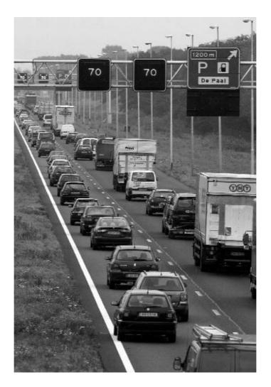
Figure 2.3: A variable speed limit gantry on the A1 freeway in The Netherlands.
